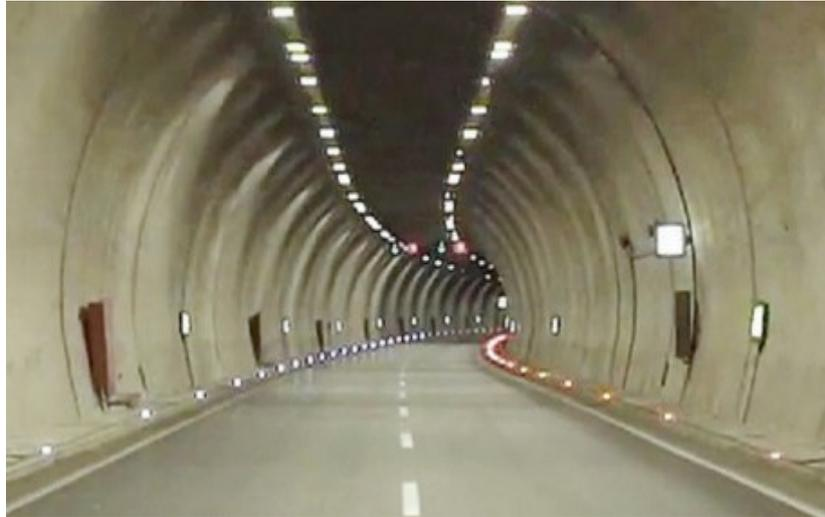
Fig. 3. A sample of tunnel LED lighting with double suspensions.
